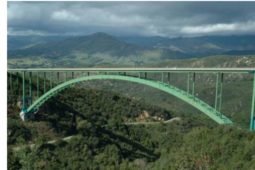
Steel 210/371m Cold Spring Bridge USA 1963
