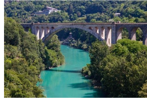
Stone 85/220m Solkan Bridge Slovenia 1906
